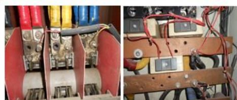
Connections without lugs
